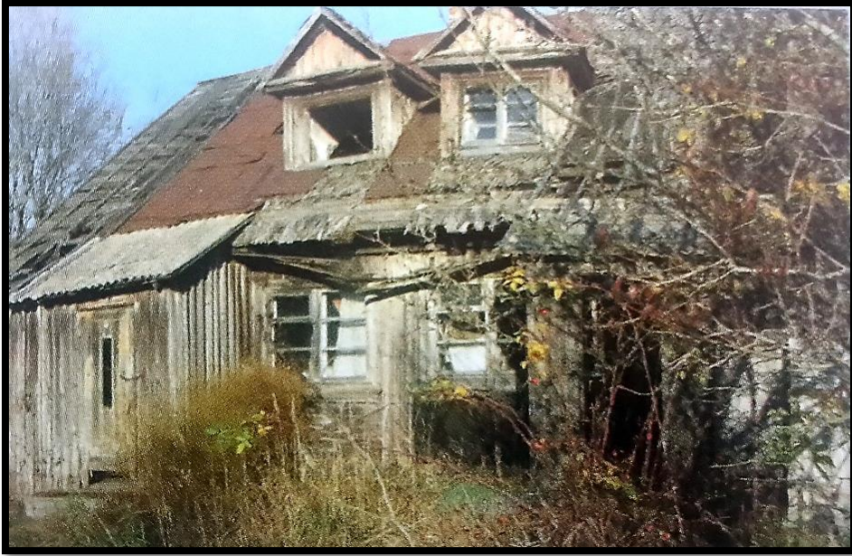
The only remaining workers house (barrack) in 2011. Today (2017) - a modern, completely rebuilt house. The picture from "Pärandkultuur Sõmeru vallas" 2014. I. Pikkoja, M. Simkin
